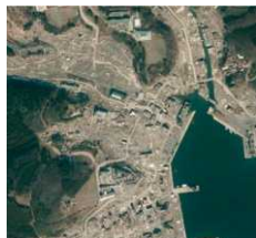
After earthquake disaster (image taken on March 19, 2011)
